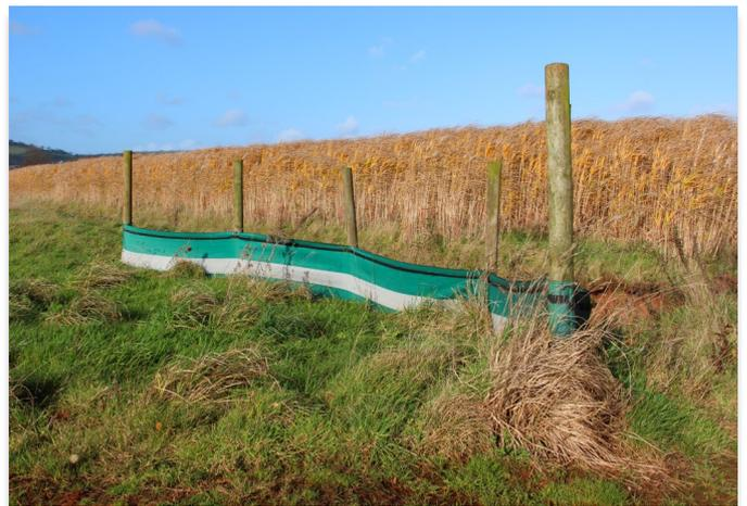
**Filter Fence** geotextile can be attached to fence posts
