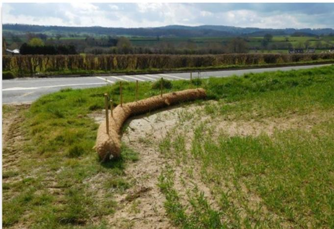
**Coir Rolls** are made from the waste coconut husks. They are relatively easily to move and install.
